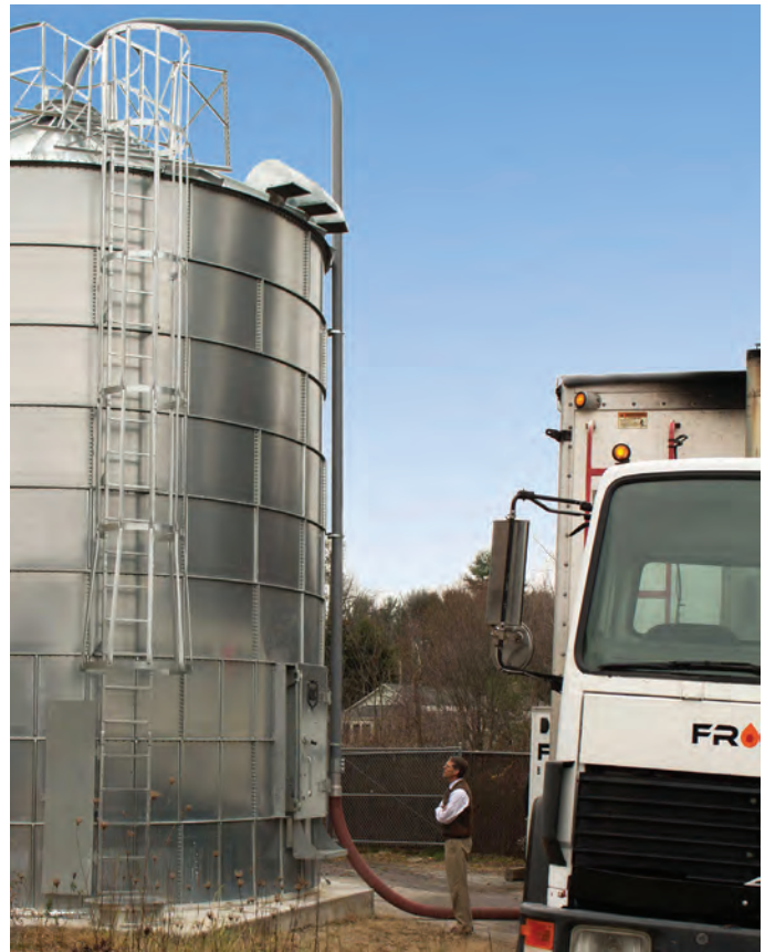
This wood chip silo is part of the John Stark High School's biomass heating facility.
