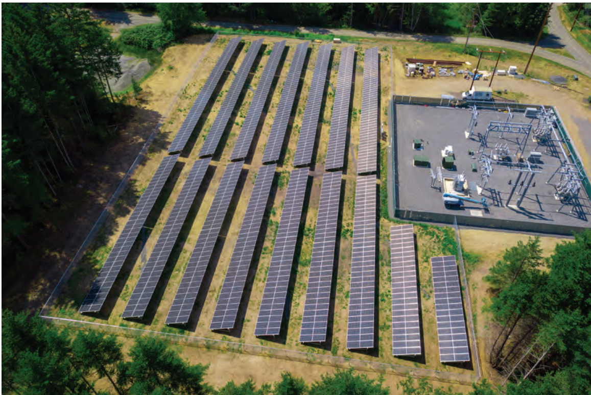
An aerial view of the Orcas Power and Light 504 kW Microgrid and Community Solar Array on Decatur Island. With assistance from a Clean Energy Fund grant, Orcas Power and Light Cooperative will procure an additional 500 kW/2.0 MWh energy storage system and controls to support multiple use cases and allow the system to operate as an islandable microgrid capable of sustained operation during system outages.
