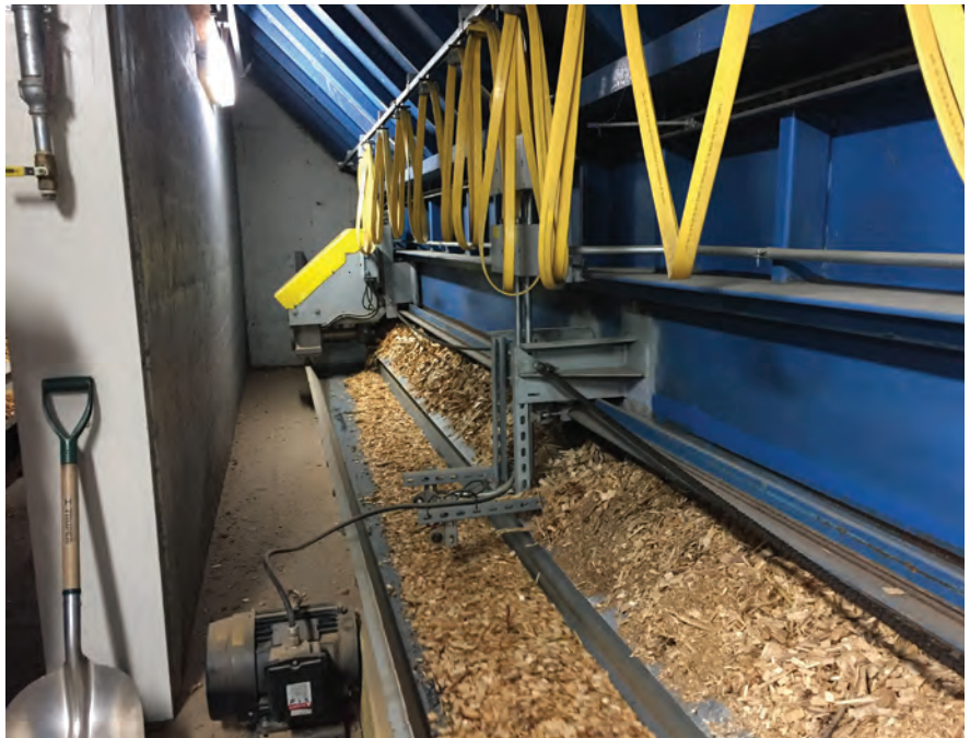
Wood chips make their way on a series of conveyer belts to Montpelier's biomass district heating system. The system provides heat to 21 buildings including the Capitol Complex, city buildings, school buildings, and private customers. The 10 MMBtu/hr project was funded with support from the Vermont Clean Energy Development Fund.
